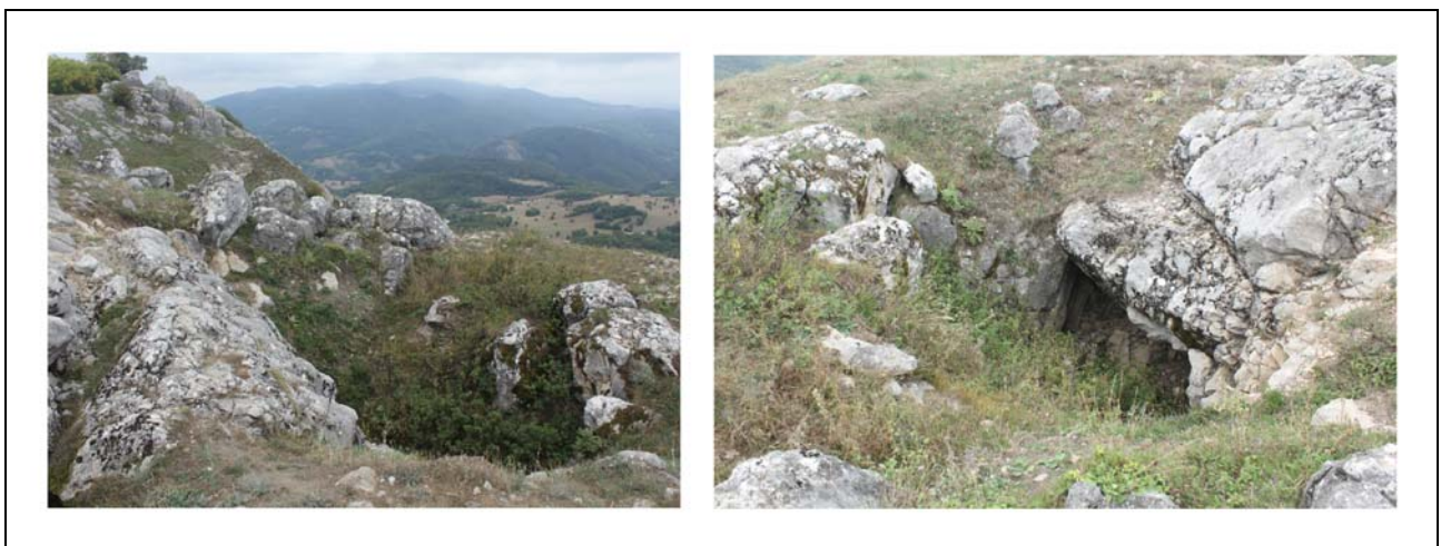
Fig. 21—22. Entrance to the damaged step tunnel.
