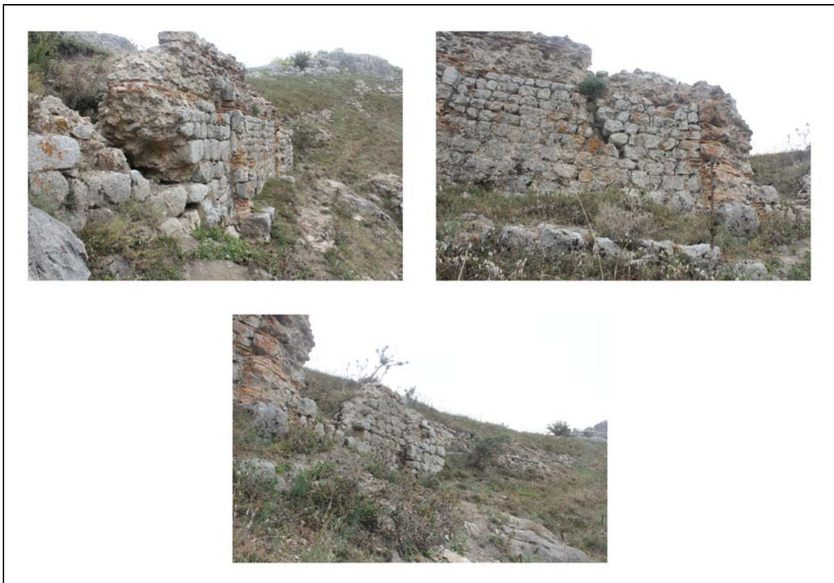
Fig. 17—19. Late-period fortifications built on the Hellenistic Period fortification walls.
